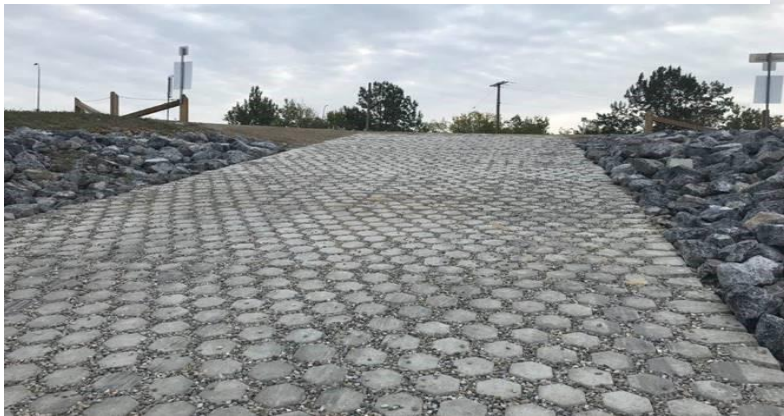
Figure 2: Calgary Ogden Bridge Boat Ramp
